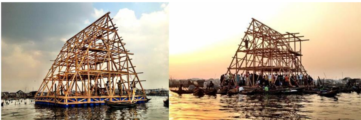
Figure 4. Structural framework, (as community gather to test the building stability) (source; www.dezeen.com)
