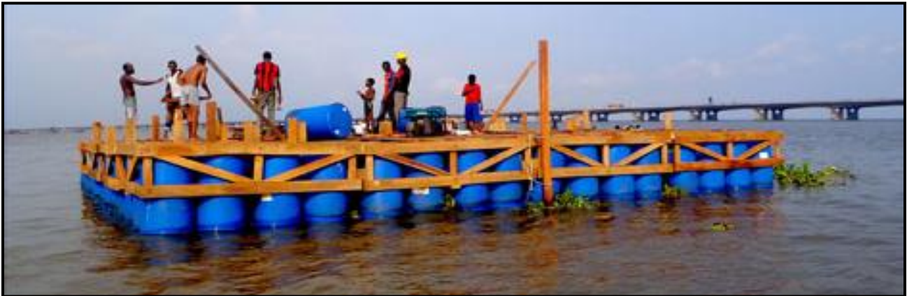
Figure 6. Base of the building during construction ( Flotation platform ) (source; www.dezeen.com)
