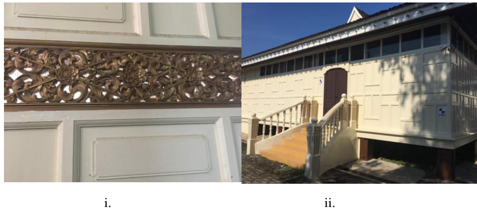
Figure 2. i) Carved timber panel and, ii) timber panelled wall at rear facades of Istana Balai Besar
