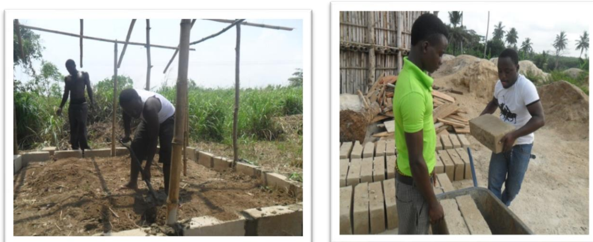
Figure 3 and 4. The youth constructing the farm house
