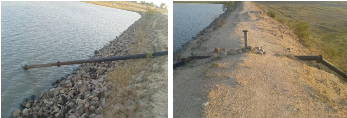
Figure 5. The syphonage system of water abstraction at Mutorahuku dam in September 2014
