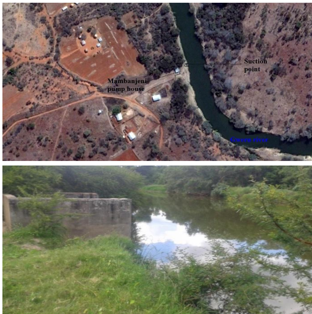
Figure 4. Plinth and pump house at Mambanjeni built on the river bank
