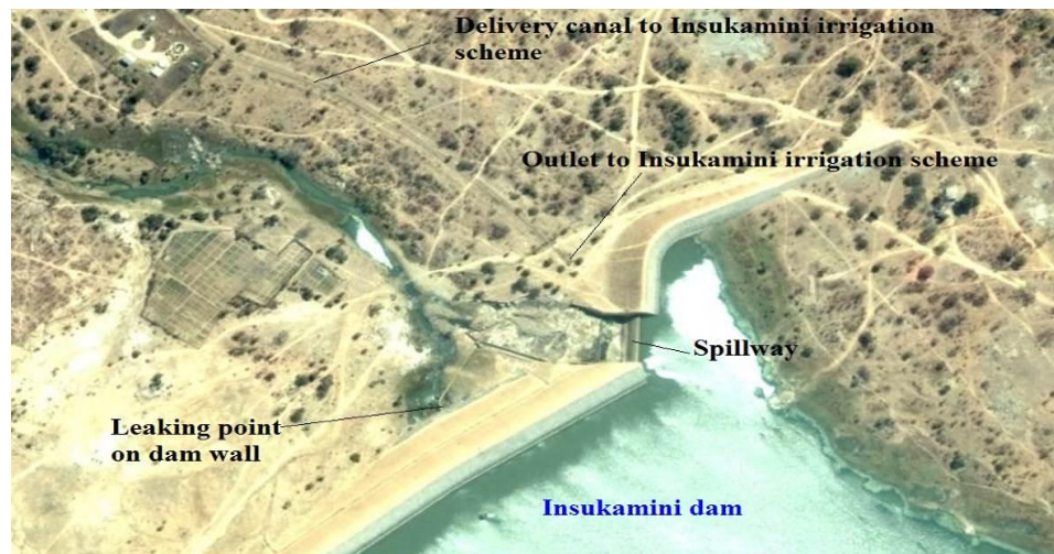
Figure 6. Insukamini leaking dam wall
