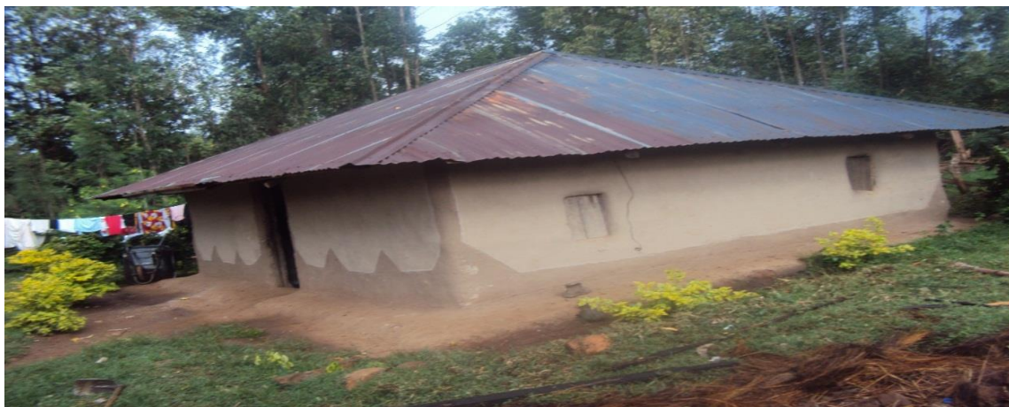
Figure 3. Wall plastered with clay near Kianjogu site at Kianjogu sub location, Meru County, Eastern Kenya
