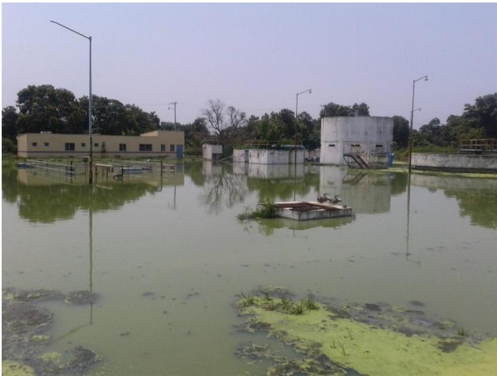
**Figure 1.** Abandoned wastewater treatment plant in the municipality of Ciuhuatlán, Jalisco. The wastewaters are still collected in an extemporary pond flooding the WWTP.
