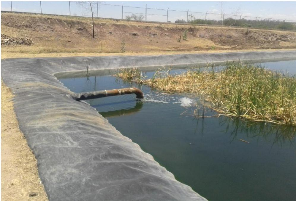
**Figure 6.** Treatment system with operational deficiencies installed in a rural community in the municipality of Teocaltiche, Jalisco. The system is based on a septic tank and artificial wetlands.
