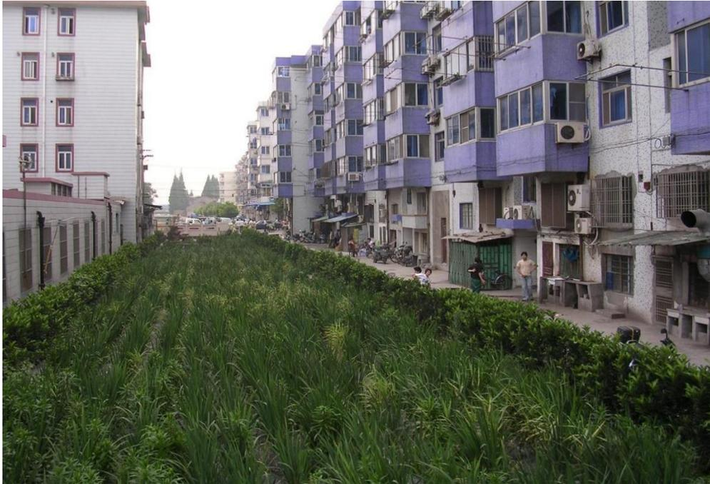
**Figure 5.** Wastewater treatment system based on anaerobic processes and artificial wetlands in Huaxin, Shanghai, China (Courtesy of Janisch & Schultz).
