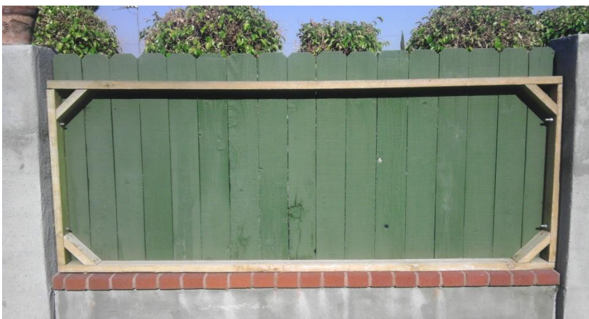
Old wood fence fitted in a new application. The panels and the studs were from a previous old fence. Recycled paint was also used (Photograph by author).
