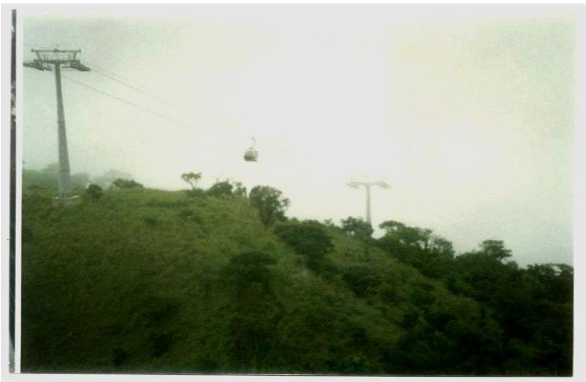
Figure 4. A Cable Car in-between the Longest Span of 1.4 km on its way up the Plateau
