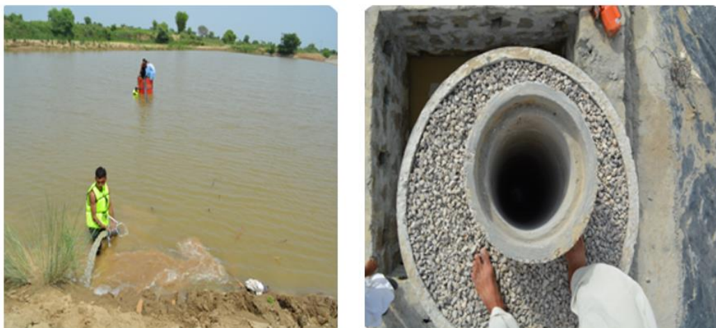
Figure 9. Water pump through indigenously designed water filter, operated through solar power system
