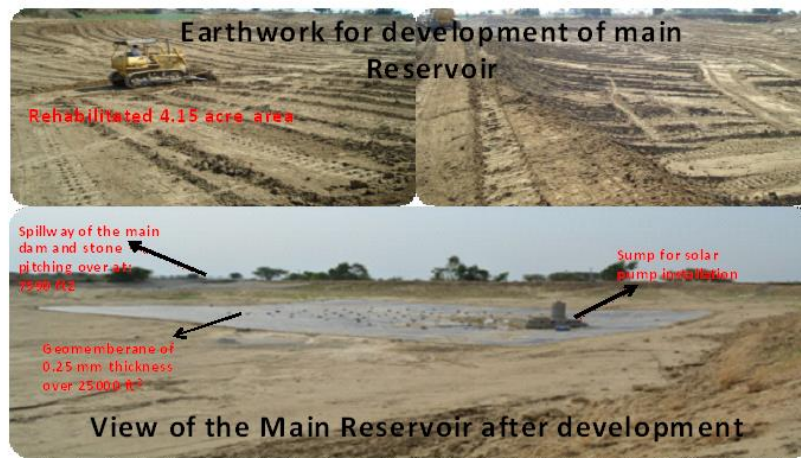
Figure 5. Showing various earth work activities at main water storage reservoir
