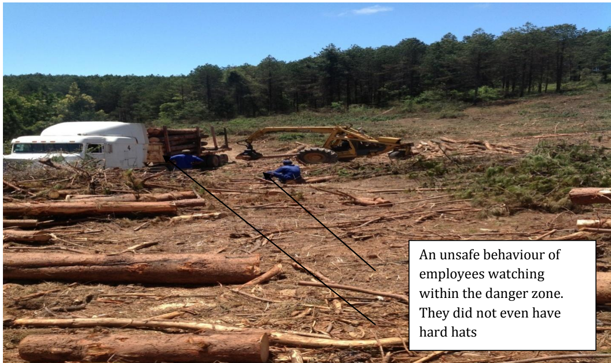
Plate 2. An unsafe behaviour of employees watching within the teler logger equipment's danger zone (Source: Fieldwork)
