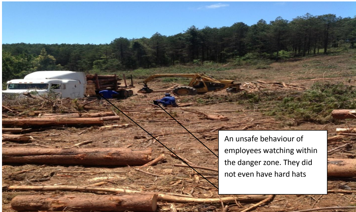
Plate 2. An unsafe behaviour of employees watching within the telle logger equipment's danger zone(Source: Fieldwork)
