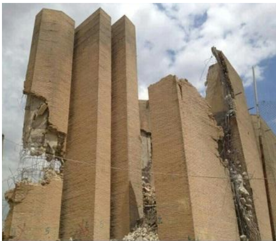
Figure 18. Demolishing the Gate in 2013
