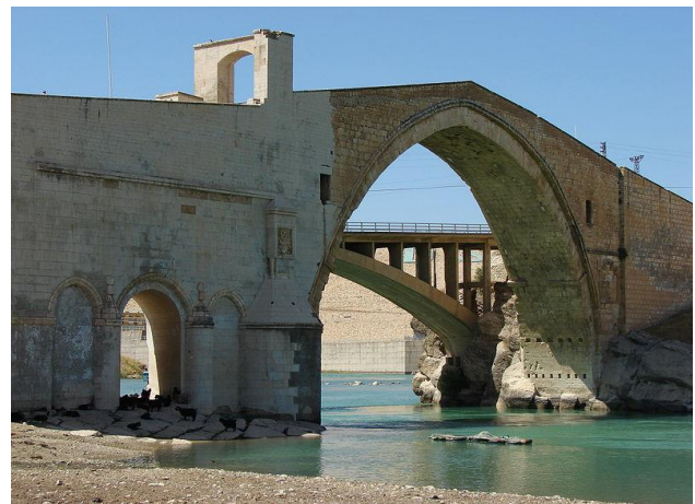
Figure 11. Bridge Malabadi, Diyarbakir Turkey 12 th century
