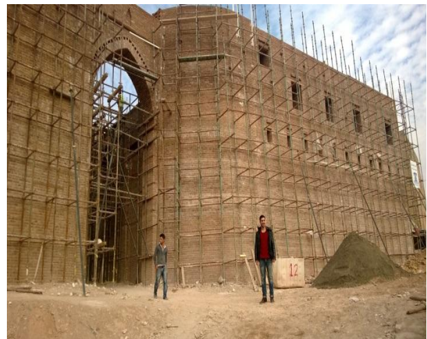
Figure 19. Rebuilding the original Gate in 2013-2014
