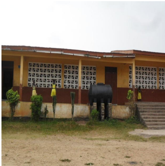
Plate 2. The condition of the School
