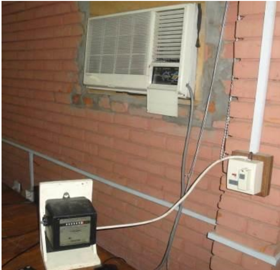
Figure 1. Metering of Airconditioner
