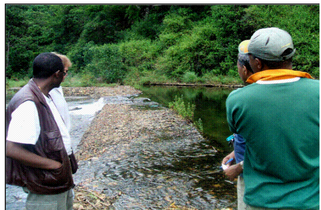
Figure 4.3. Gabion dam structure at the head of the valley
