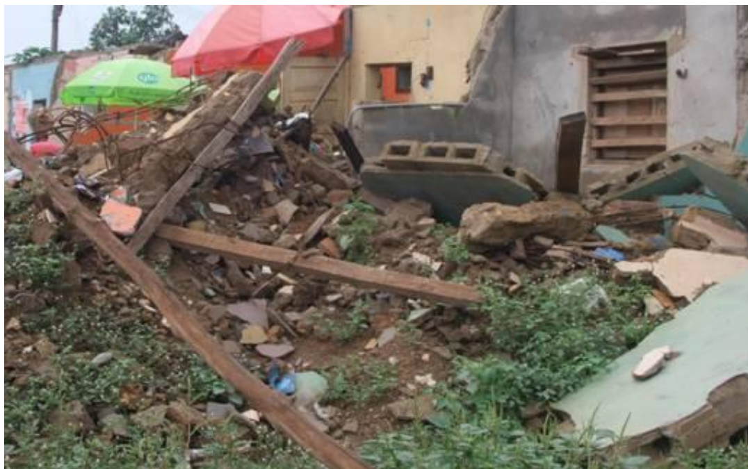
Figure 1. A demolished building around state hospital road in Ado-Ekiti, Ekiti State, Nigeria
