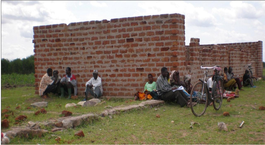
Figure 2. Unfinished School building in Mwabujiku Village
