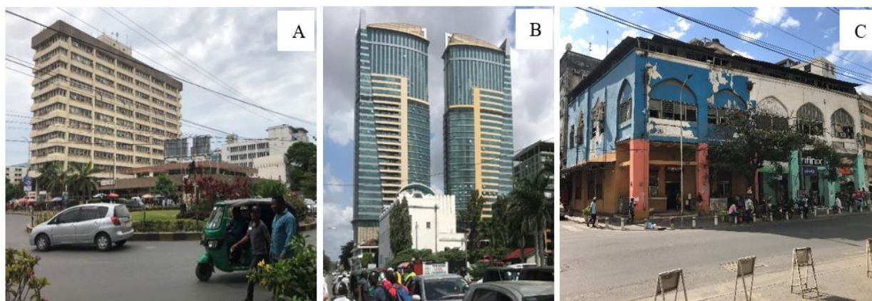
Figure 2. A - The IPS building, B - PSSSF Twin Towers, and C - the HOSCO building (Source: Author, 2021)
