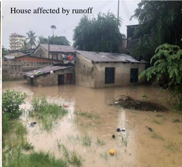
Plate 2. Flooded house during rainy seasons (Source: The Presidents' Office-Regional (PO-RALG), 2020)
